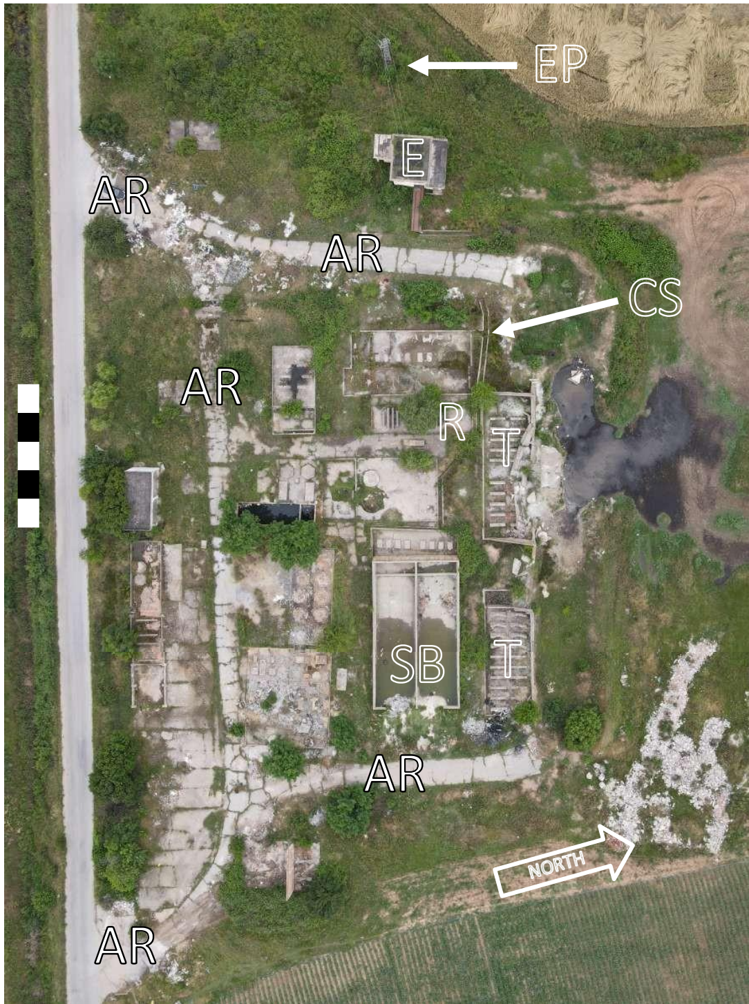
Fig. 4. Momino ISL site along the road from Rakovski to Momino Selo. Some of the identified features are labelled: AR = access road; CS = canal structure; E = electrical supply building; EP = electricity pylon and supply cables; R = ramp; SB = separation basin; T = site for storage tanks. This has become a popular site for dumping rubbish – see by the “North” arrow for example. Scale bar on left margin = ca. 25 m, each subdivision = ca. 5 m. Arrow points to the North. Drone (UAV) photograph, June 2021.
