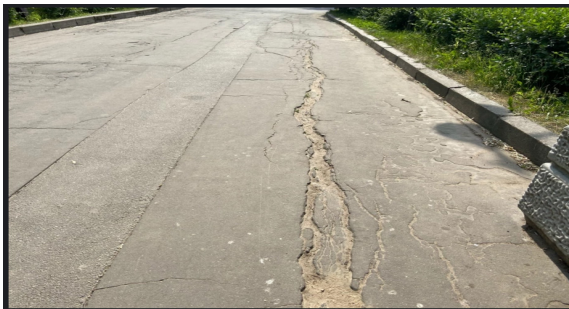
Figure 10. Example of cracks in the asphalt concrete pavement of a park area
