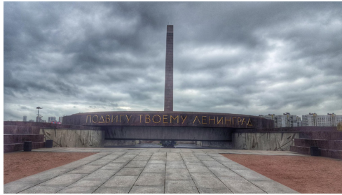
Figure 3. Architects Speransky S. B., Kamensky V. A. Memorial to your Feat Leningrad
