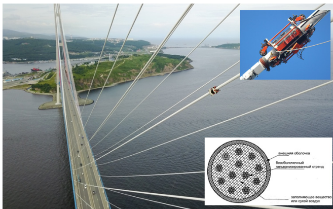
Figure 3. Moving the INTROS flaw detector (MG 120-300) along the cable stay of the PSC bridge to Russky Island (Vladivostok)
