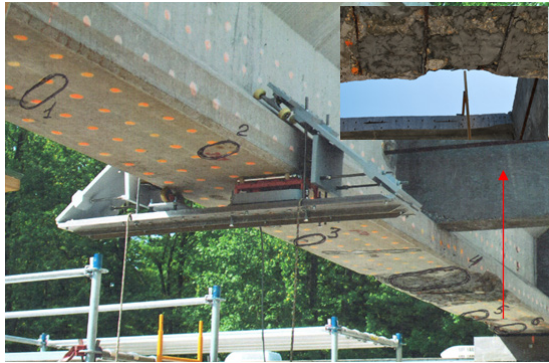
Figure 11. Bridge beam inspection section
