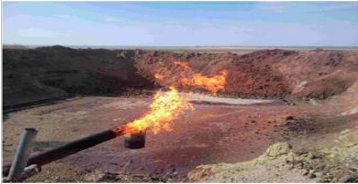
SHYRAK-1 WELL GAS FLARING DURING DRILLING
