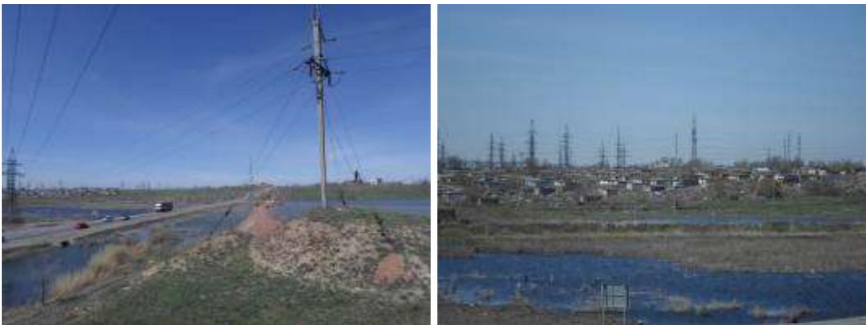
Figure 2 - Destruction of garages and the M36 highway near the mined areas
