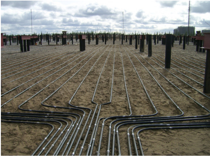
Figure 1. General look of a horizontal soil collector
