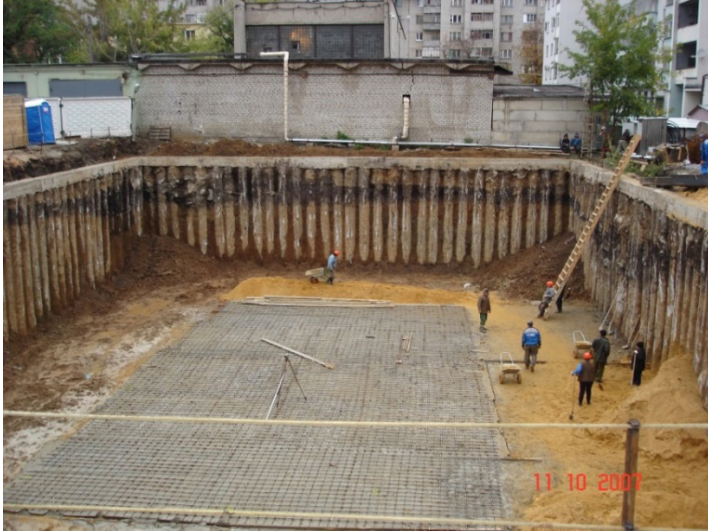
Figure 4. General look of the foundation wall with thermal probes
