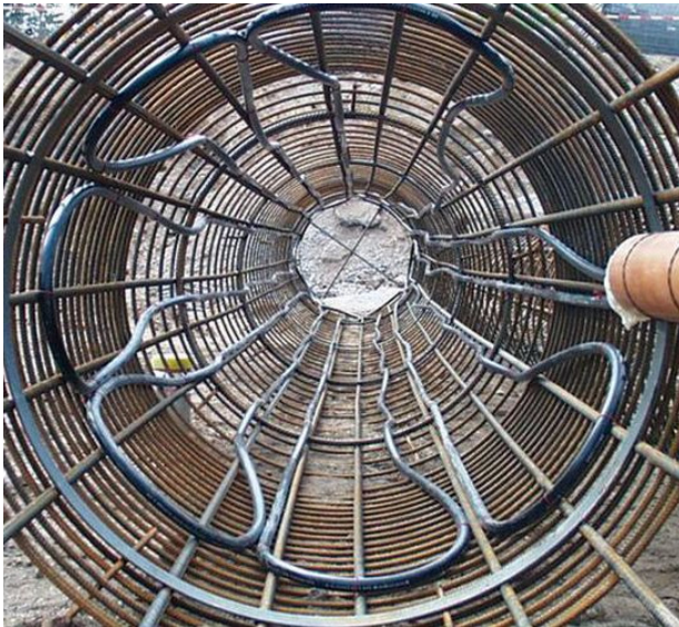
Figure 3. General look of the pile frame with thermal probes
