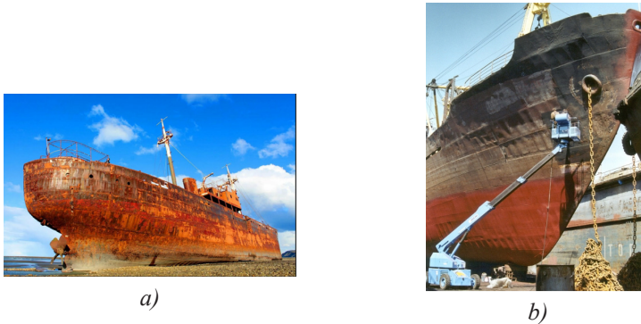
Figure 5. Rusty ship (a); application of paint and varnish coatings to the vessel.
