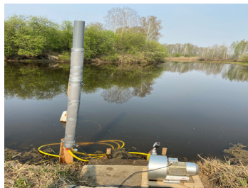
Figure 7. Photos of a model experimental installation for obtaining cold with an intermediate heat exchanger.
