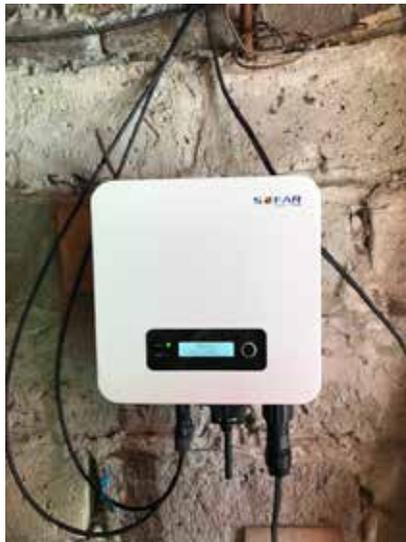
**Figure 2 – Installed Sofar inverter**
