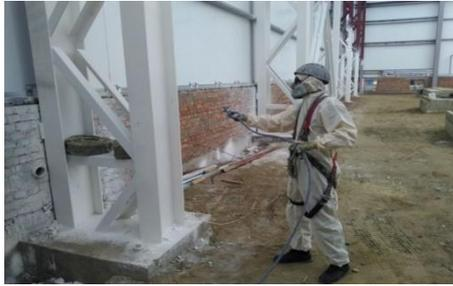
*Fig.4. The infliction of thick-layer fire-resistant covering*
